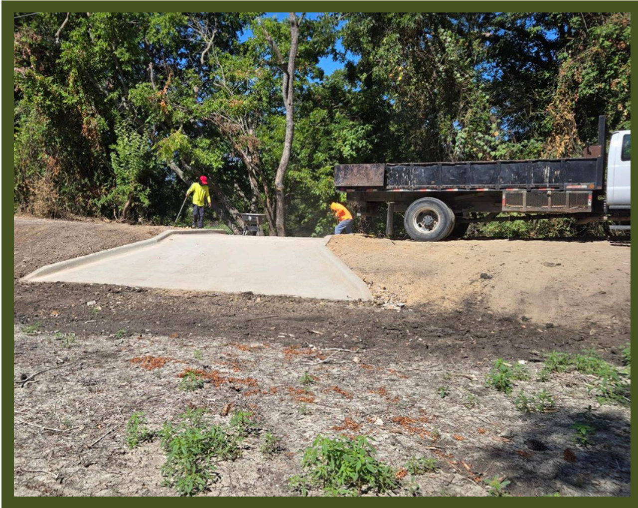
JEWEL PARK DAM AND SPILLWAY REPAIR
