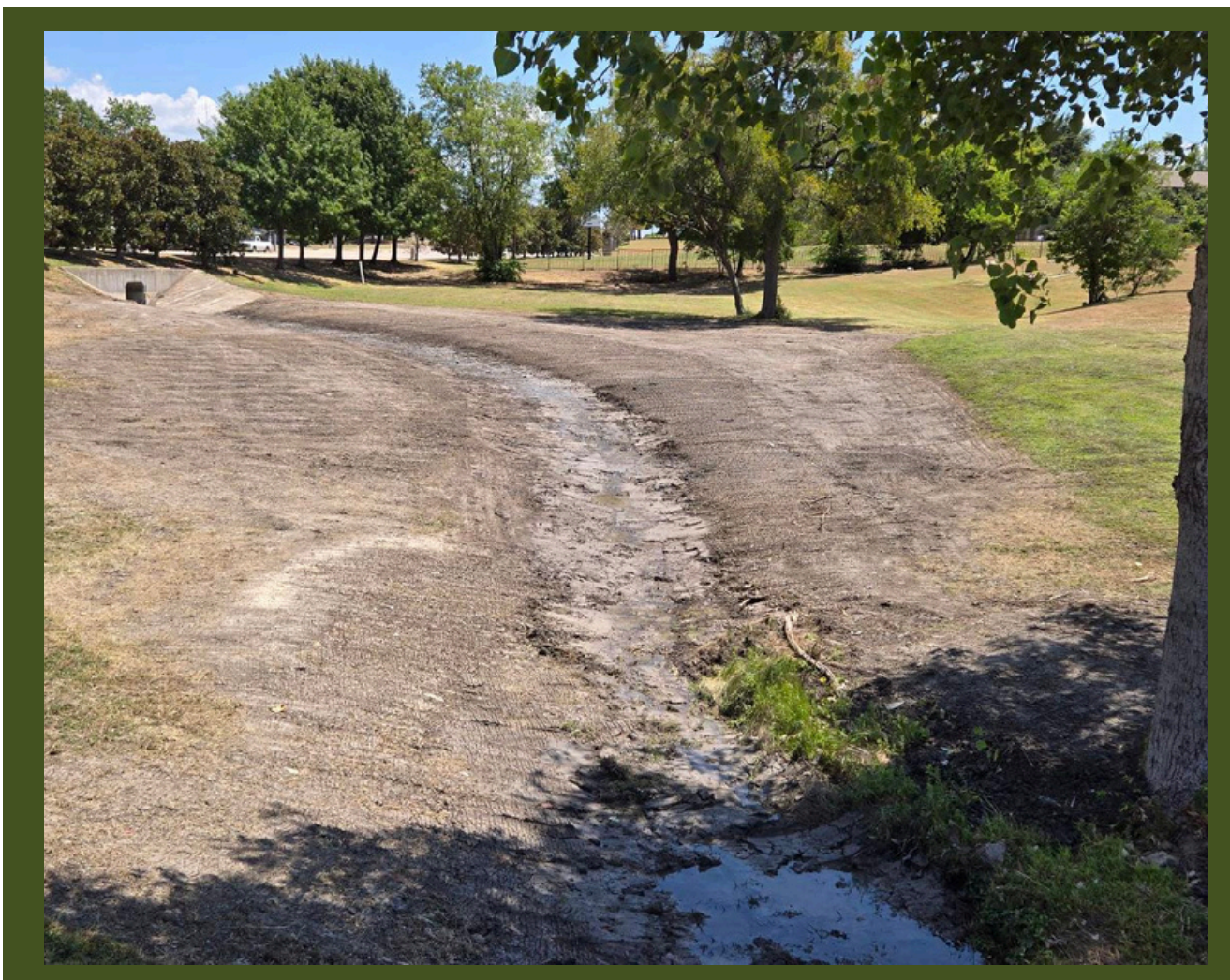
205 CEMETERY DRAINAGE REPAIRS
